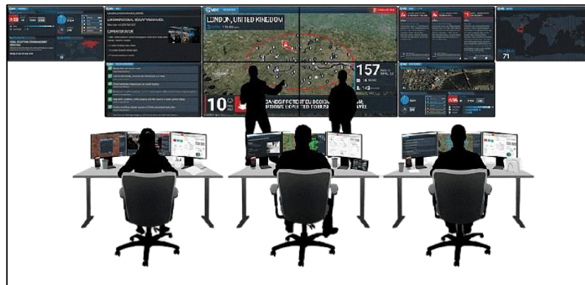
Figure 36: A view of a Control Center
